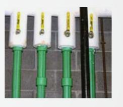
Thermal Insulation of PPR tubes at roof Plumbing
